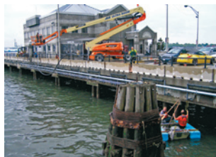
Final attachment of the pipe to the pier
