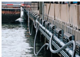
Temporary attachment of the pipe
