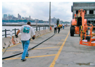
Deployment of 500 ft. of FLEXWELL®-HL pipe
