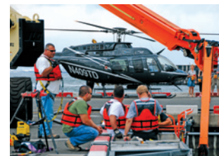
Installation work during ongoing helicopter traffic
